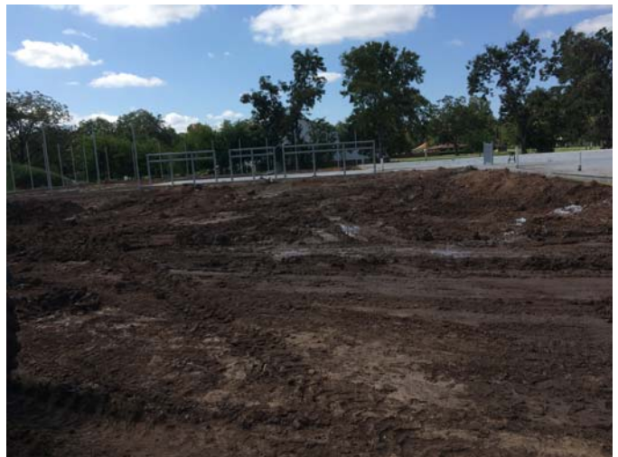
6. Rough grade after concrete for removal
