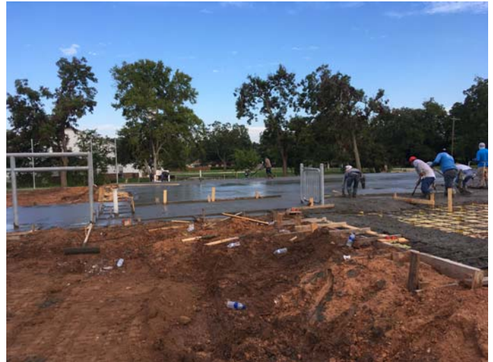
4. Concrete finishing at slab on grade
