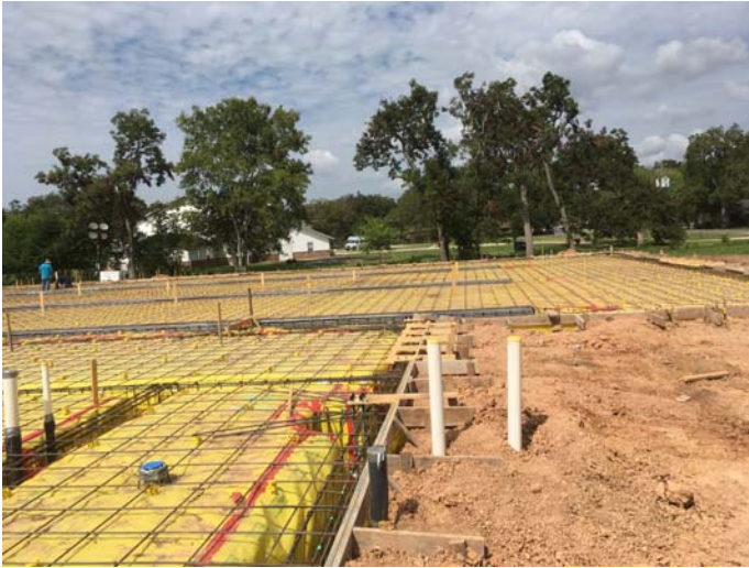
1. Concrete prep at reinforcing steel
