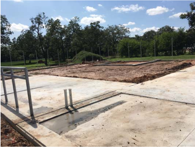
7. Concrete foundation at wash down area
