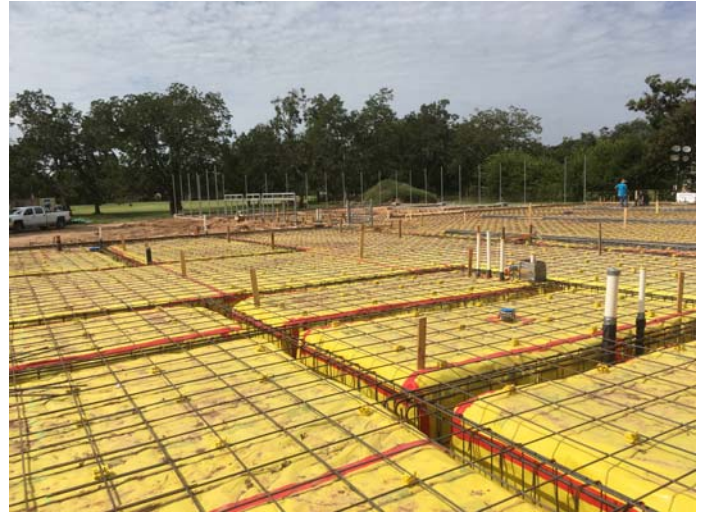
2. Concrete prep at reinforcing steel
